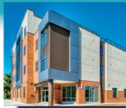
Project HOME Gloria Casarez Residence
